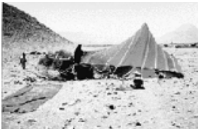
Hassaniya tent. South West Morocco: airfoil design for the desert winds. Photo: Peter A. Andrews.
