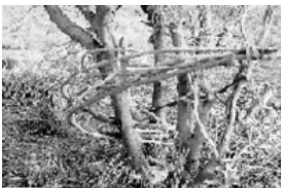
Fabrication of bent acacia arches. Northern Kenya. Photo: Labelle Prussin.
